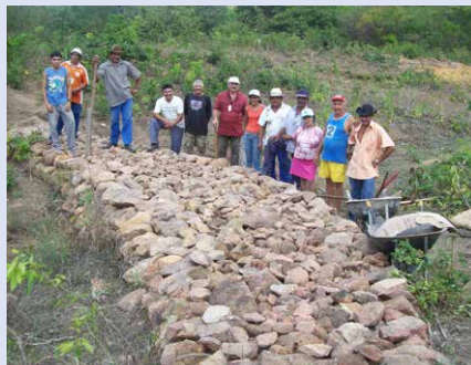
Photograph 02 – Collective activity for construction of succession dam
