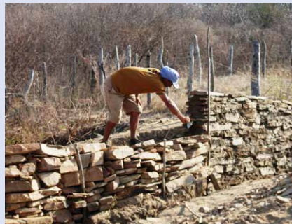
Photograph 02 – Construction of dry stone dam
