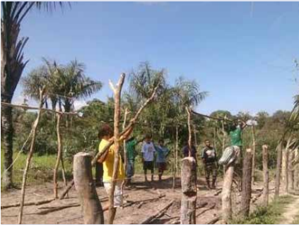
Photograph 01 – Plant nursery construction
